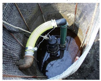
a 110 volt pump because of the reduced current and voltage drop. In our demonstrations, sewage pumps operated well even with voltage drops up to twice the generally recommended limits. In some cases, a second pump might be recommended to add system capacity and reliability while keeping the cost down.
