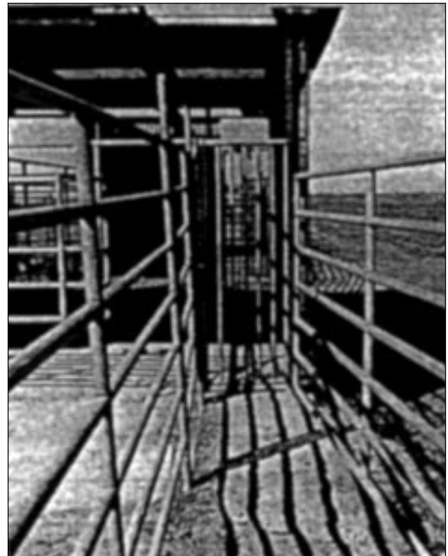
Figure 1. Poorly designed chute with open bar sides. Solid fences will eliminate the shadows formed by the bars.
