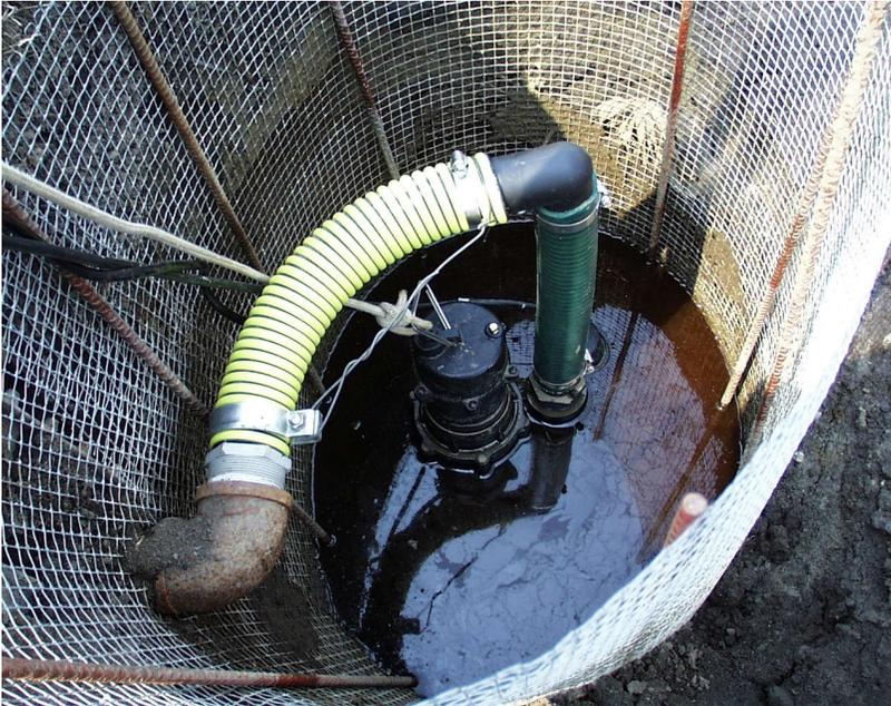
Most sewage pumps provide less than 20 feet of lift capacity. If the topography to the field requires more elevation lift, make sure to select a pump that can deliver.
